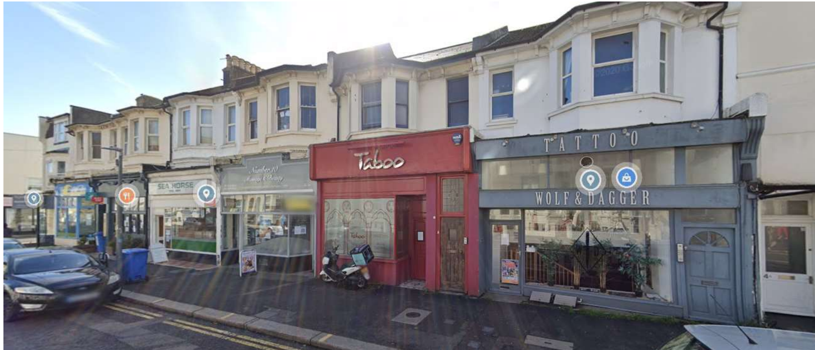
Application site is 'Taboo' with the red shopfront. (Google, October 2020)
