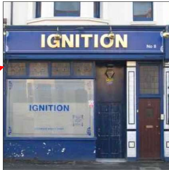
Image 1 - Former Shop frontage (reinstated upper stained glass windows as part of proposed shop frontage)
